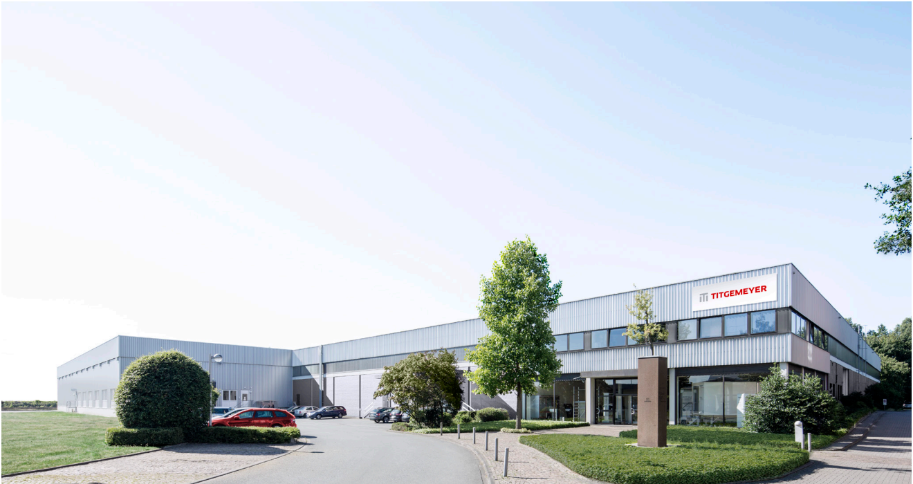
Das Zentrallager in Osnabrück
